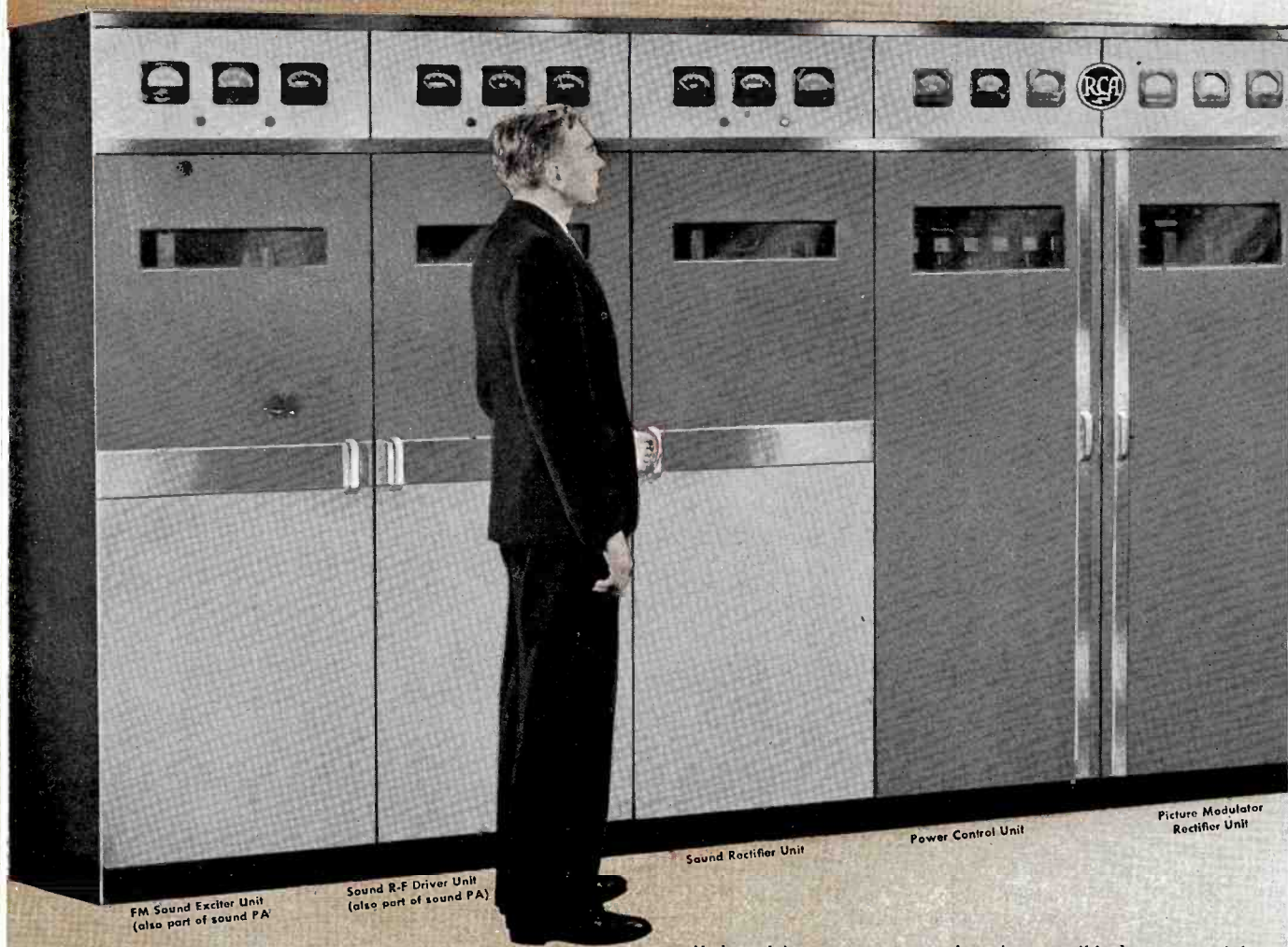
Straight-line Arrangement (over-all width, 208 inches). Unit-construction permits flexible station layout, advantageous use of available floor space.
